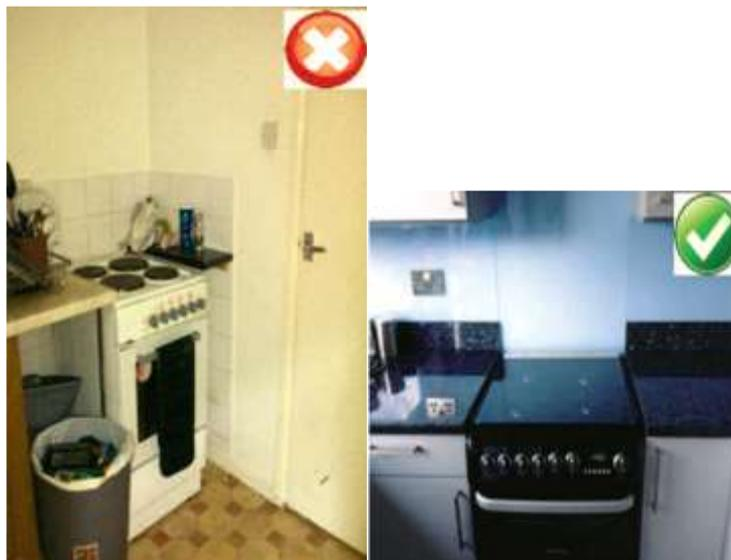
This cooker location meets the minimum requirements for a suitably sited cooker with sufficient worktop to both sides of it.
