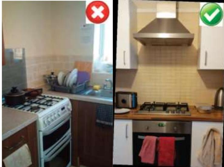
This layout meets the minimum requirements as there is adequate worktop to both sides of the cooker and suitably located extraction.
